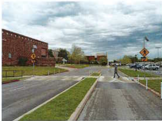
Rectangular Rapid Flashing Beacons
