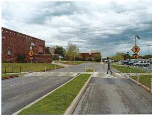
Rectangular Rapid Flashing Beacons
